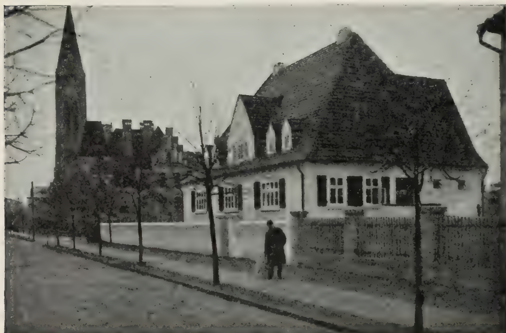
DR. DISCHLER'S HOUSE AT SWINEMÜNDE PROF. PAUL SCHULTZE-NAUMBURG, ARCHITECT
